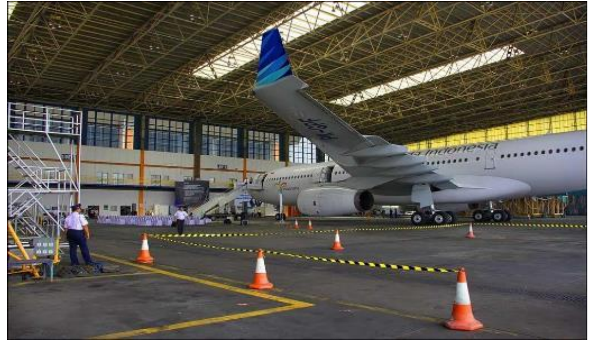
Garuda Indonesia Maintenance Facility
